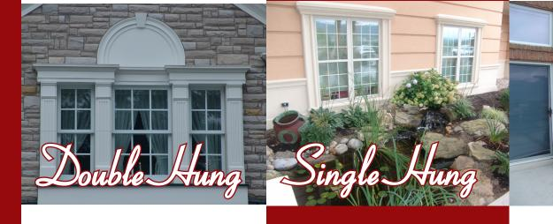
Double Hung windows are best suited to traditional Single Hung windows are also best suited to tradiarchitectural styles. Both sashes on a double hung win- tional architectural styles. The lower sash on a single dows slide vertically past each other and tilt in for easy hung window slides vertically past and tilts in for easy cleaning.
